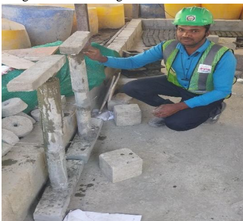
Figures: Pier casting for erection of Slab.
