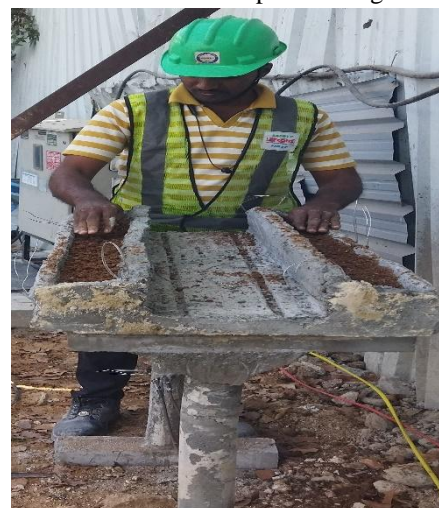
Figures: Slab erected and soil placed for green forestry.
