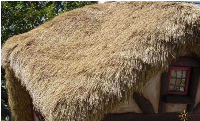
Figure 1 Roof Covering Material
