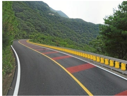
Fig. 1 Rolling barrier in hilly area
