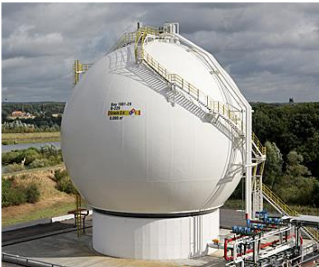
Fig. 1.2 Spherical Pressure Vessel
