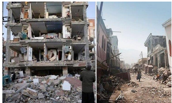
Fig.1: Failure of Buildings Due to Earthquakes
