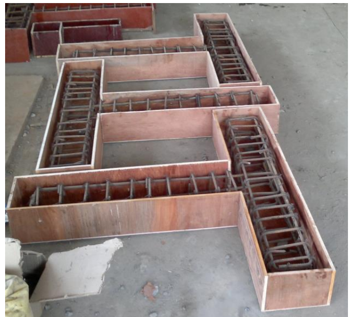
Figure 4.1 Wood Cum Reinforcement
