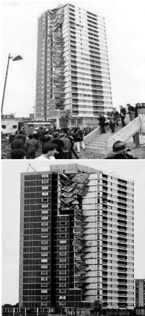
Fig. 1.1: The collapse of a part of the Ronan point apartment
