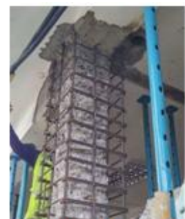
Fig.2. Additional Reinforcement
