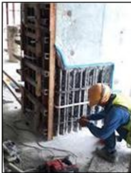
Fig.4. Concreting with micro concrete
