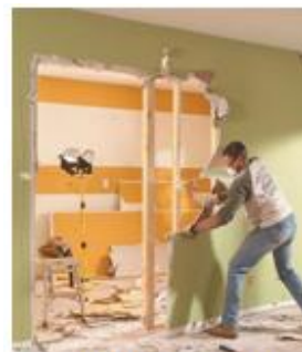
Fig.1. Removing brick work
