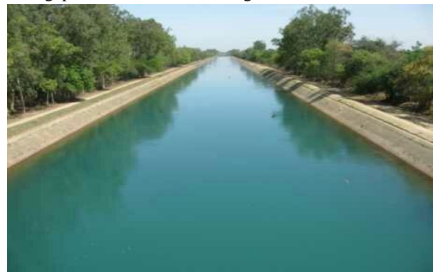
Fig.3.1 Pictorial view of Gangapur Canal
