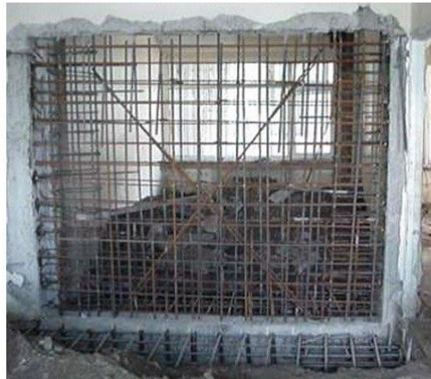
Fig 1.2. Additional Shear Wall
