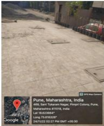
Fig4:Underground Water tank
