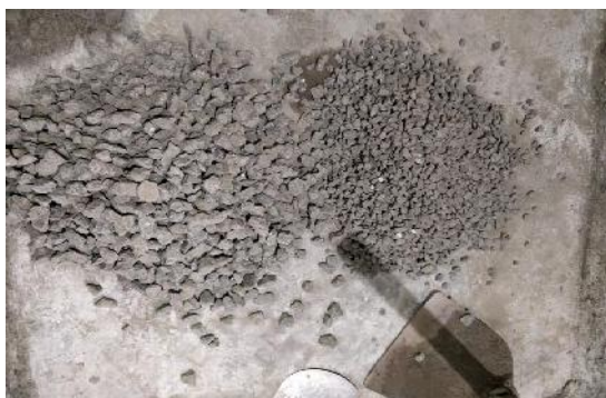
Fig 3.12 – Mixing of 20 mm and 10 mm aggregate.
