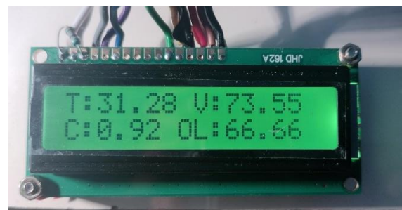
Figure3.Status of Transformer parameters
