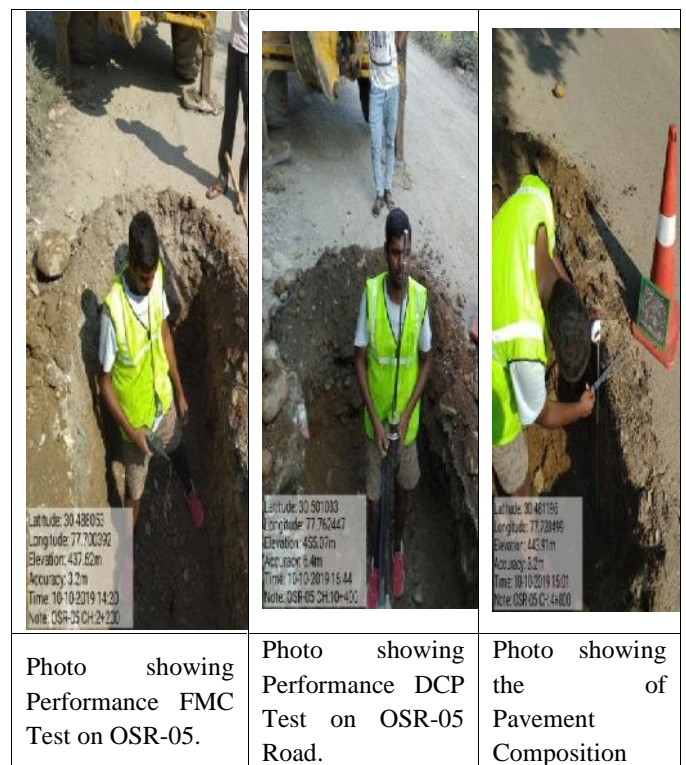
Figure 3: Photographs showing Filed Investigations along the theProject Road
