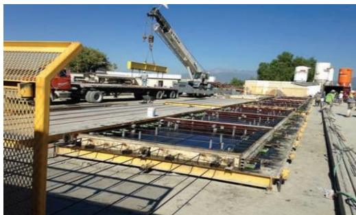
Figure 5 Photo of JPrCP fabrication in a prestressing bed.
