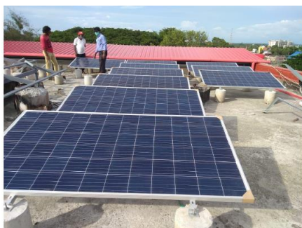
Fig. 4 Solar Modules, 325W/330Wp Multi crystalline
