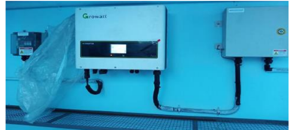
Fig. 5 Growatt Grid Connect Solar String Three Phase Inverter- 6 KW
