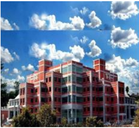
Figure:1 Hitkarini College of Engineering, first green building in Jabalpur, Certified by GRIHA.
