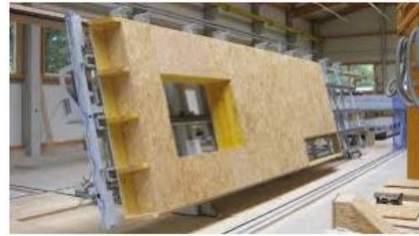
Fig 2 prefabrication In Housing Construction
