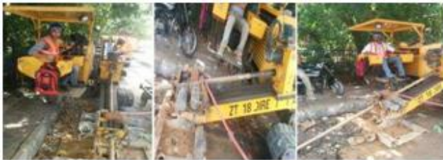
Figure 6: Pipe Ramming In KDMC
