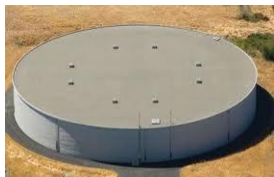
Fig No 1: . Tanks Resting On Ground
