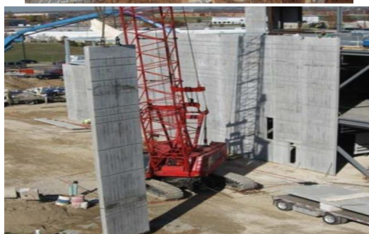
Figure 1: Precast wall panel and Installation of precast concrete wall panel
