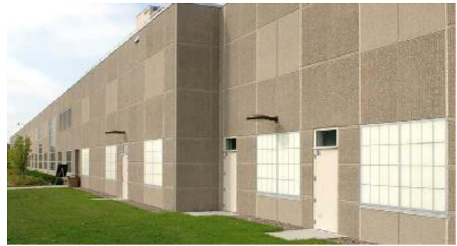
Figure 2 Precast non-composite concrete wall panel.
