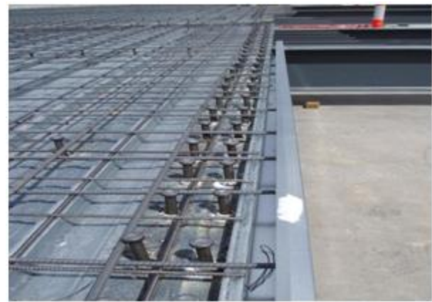
Fig 1.4 Shear Connectors
