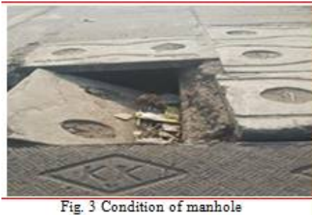
Fig. 3 Condition of manhole
