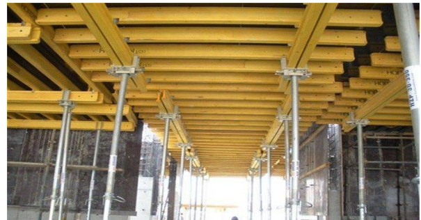
Fig 2 Shuttering of flat slab
