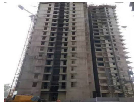
Fig- 1 Showing the Mivan technology used for the building
