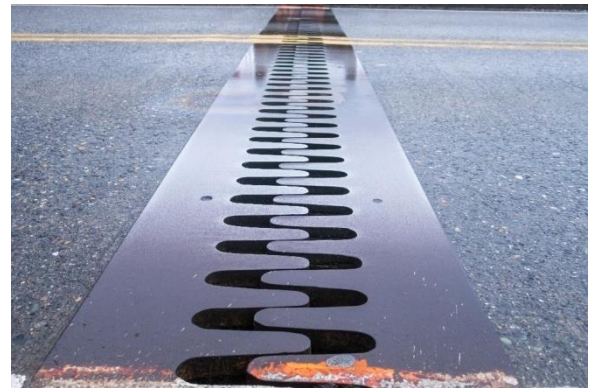
Fig. Expansion joint
