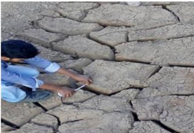
Figure 2. Expansive Soil Showing Cracks
