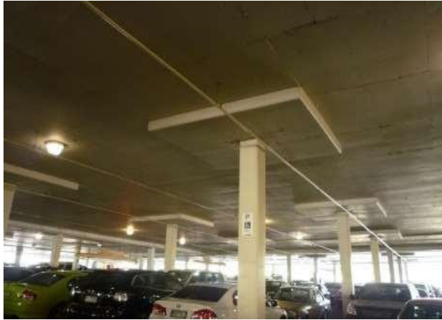
Figure 1: A Typical Flat slab
