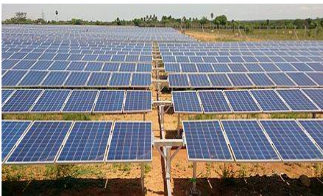
4 MW horizontal single-axis tracker in Vellakoil, Tamil Nadu
