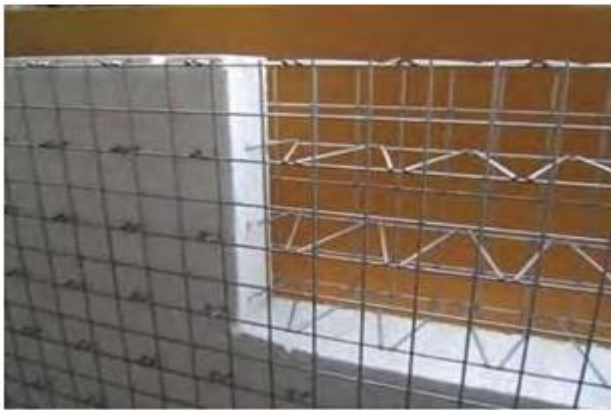
Figure 2. Reinforcing mesh expanded polystyrene core and diagonal wire.
