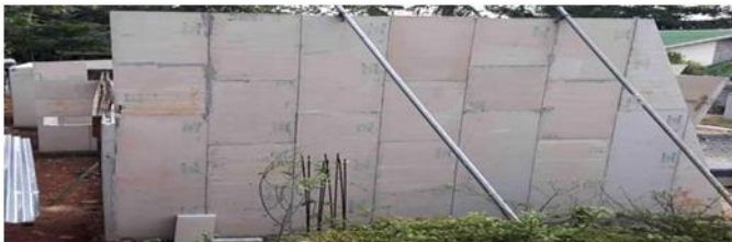
Figure 5. EPS wall panels arranged in staggered joint manner. 35 (Reproduced from Ref. 35, with permission from Elsevier.)
