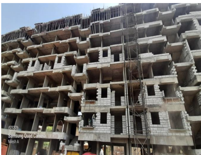
Fig – Ongoing construction at site
