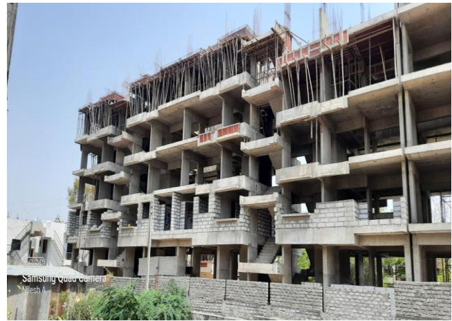
Fig – Ongoing Construction at
