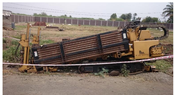
6.1 Microtunneling Bore Machine ‘Vermier series 48’
