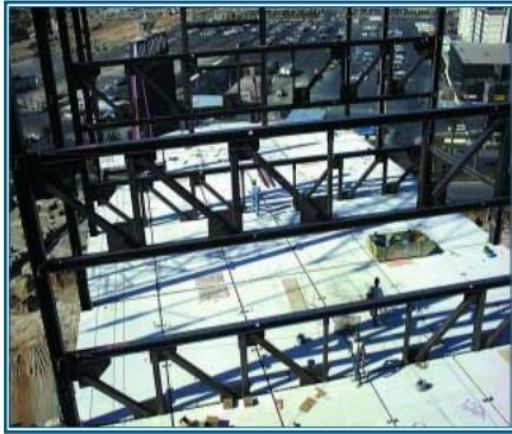
Fig .1.3 Staggered truss placed on floor
