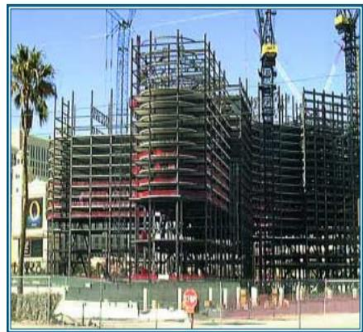
Fig .1.2 Staggered truss used in hotel
