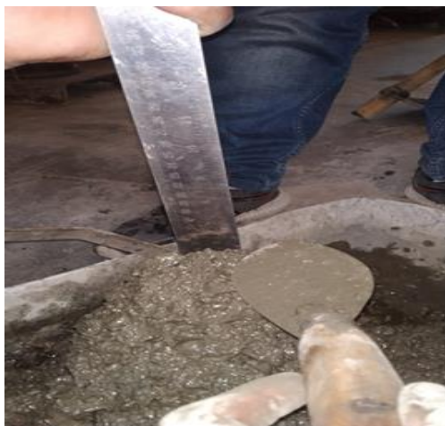
Photo. No: 1 Checking Workability of concrete
