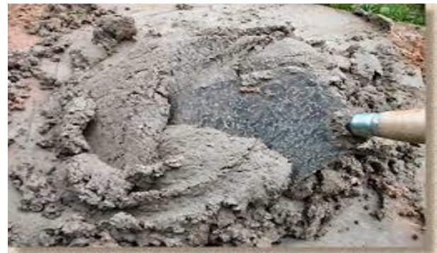
Fig1 -: Mixing of GPC materials
