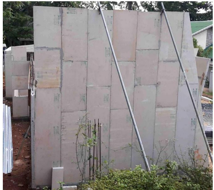
Figure 5. EPS wall panels arranged in staggered joint manner. 35 (Reproduced from Ref. 35, with permission from Elsevier.) [Color figure can be viewed at
