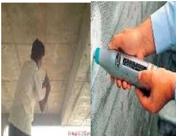
Fig 7 : Non-Destructive Test [NDT] on Column and Slab in Building
