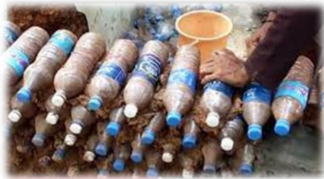
Fig. 5.3.6 Execution of work
