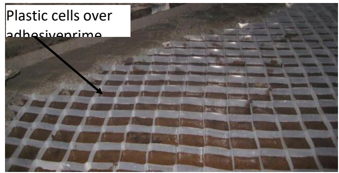
Casting of the PCCBP overlay adhesive prime coat
