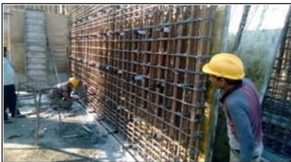
(Image: - Fixing offformwork)
