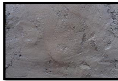
Figure 4.4.1- 0.5 % Plaster Patch withoutCracks
