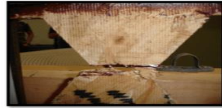
Fig-1.5 Rupture of Welded Joint
