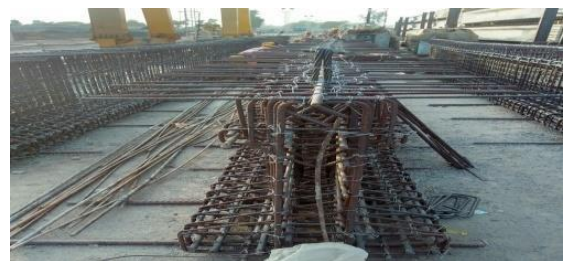
Fig.Reinforcement of I girder
