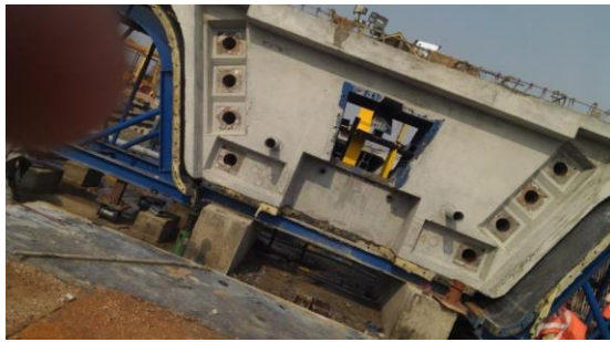
Fig. Segment of Box Girder
