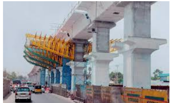
Fig.I girder platform level
