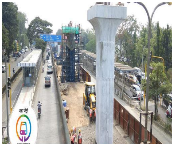
Fig.Pier at Nagpur Metro Construction Site
