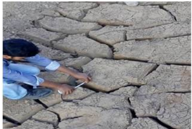
Figure 2. Expansive Soil Showing Cracks
