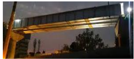
Fig 10: Composite Girder section at Ramzhoola, Nagpur
