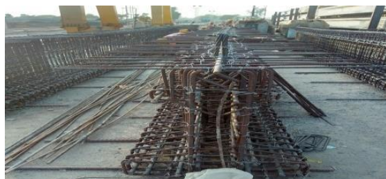
Fig 8: Reinforcement of I girder
