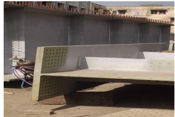
Fig 9: Composite Girder
