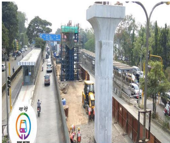
Fig 6: Pier at Nagpur Metro Construction Site
