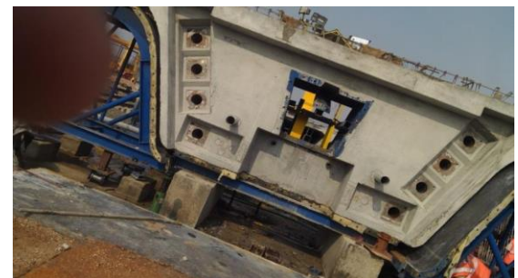
Fig 11: Segment of Box Girder
