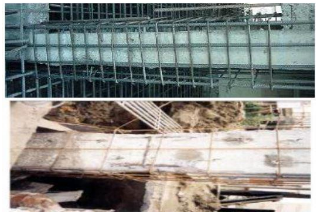
Figure: 1.4 Picture showing column jacketing
