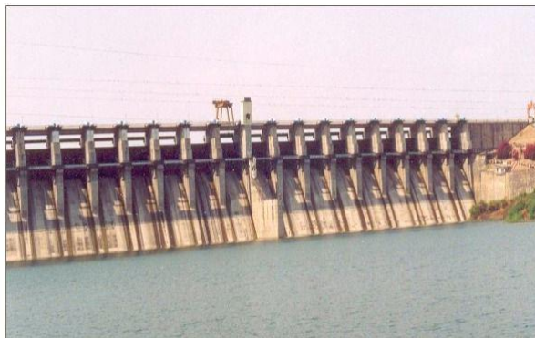
Figure 4.1: Photograph shows the close view of the Jaikwadi dam (Nathsagar Reservoir)
