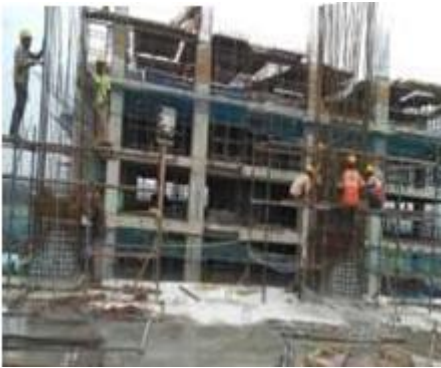
Source: Ramakrishna Venuzia Techno Towers at nearby ANU (Table formwork).
