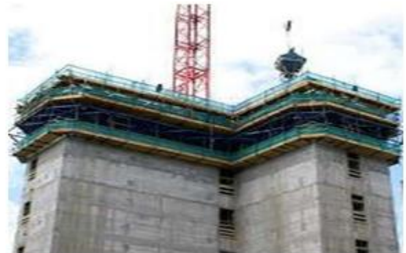
Source: Ramakrishna Venuzia Techno Towers at near by ANU.(Slip formwork)
