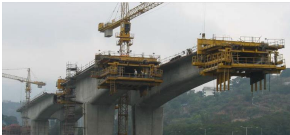
Fig -1: Balanced Cantilever Bridge
