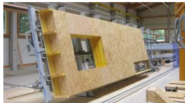
Fig 2 prefabrication In Housing Construction
